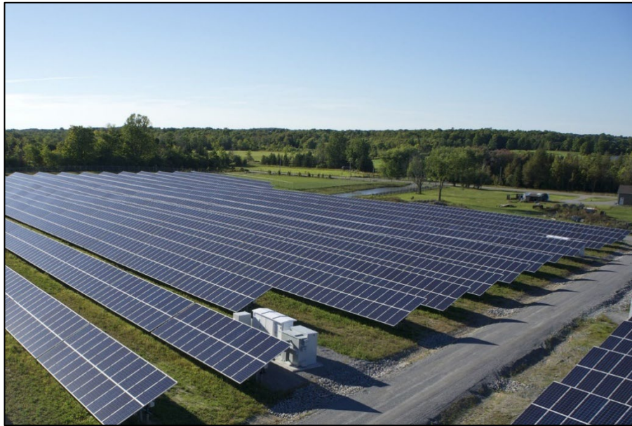
Plate 5 Typical Fixed South Facing Arrays (with Conversion Unit/Inverter)
