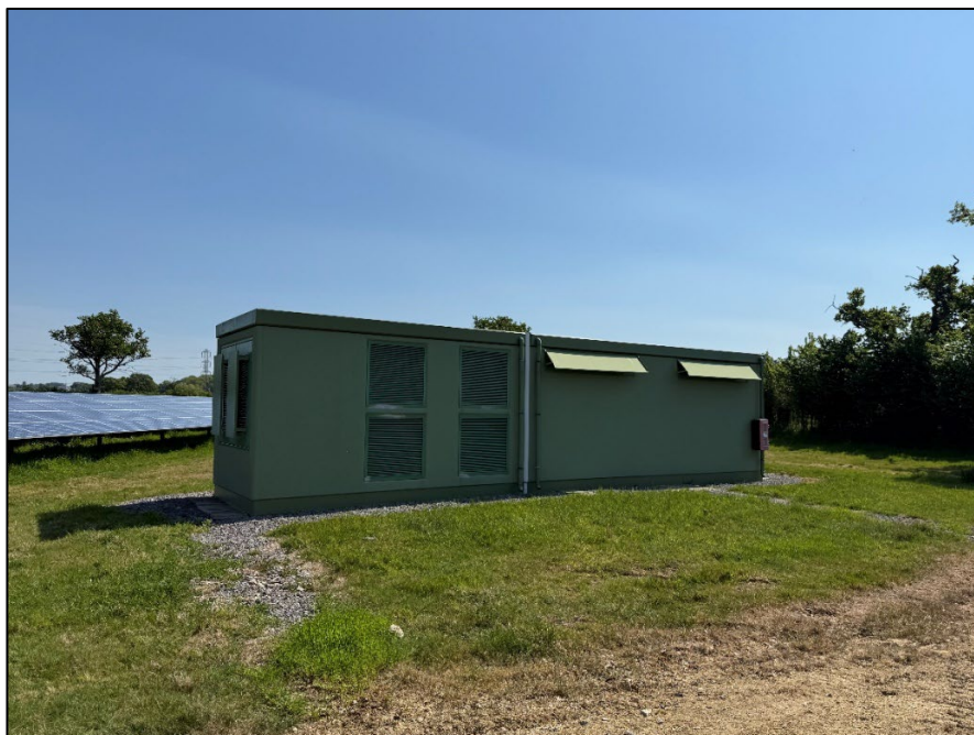
Plate 6 Typical Conversion Unit / 33kV Sub-distribution Switch Room
