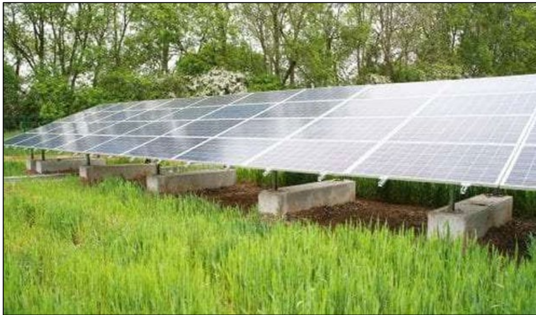
Plate 4 Fixed Panels on Concrete Feet
