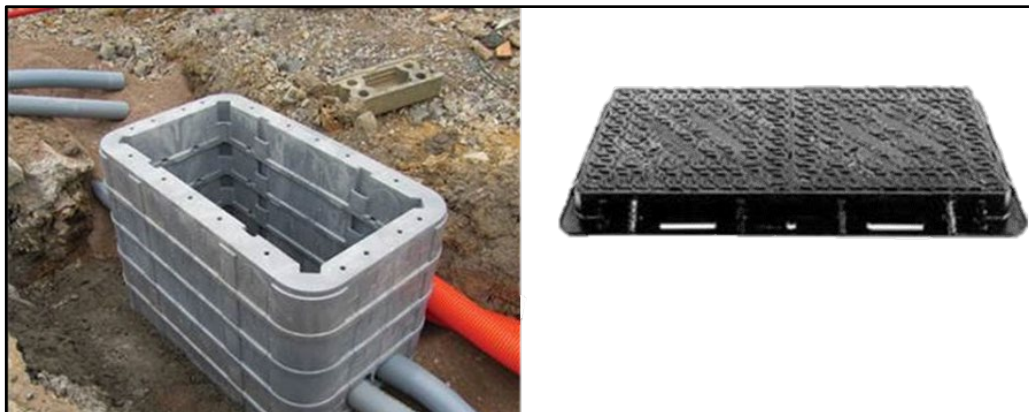
Plate 12 Fibre Chambers (construction and external appearance)
