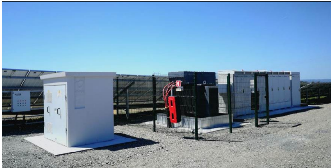
Plate 8 Typical Standalone Equipment Making Up a Conversion Unit
